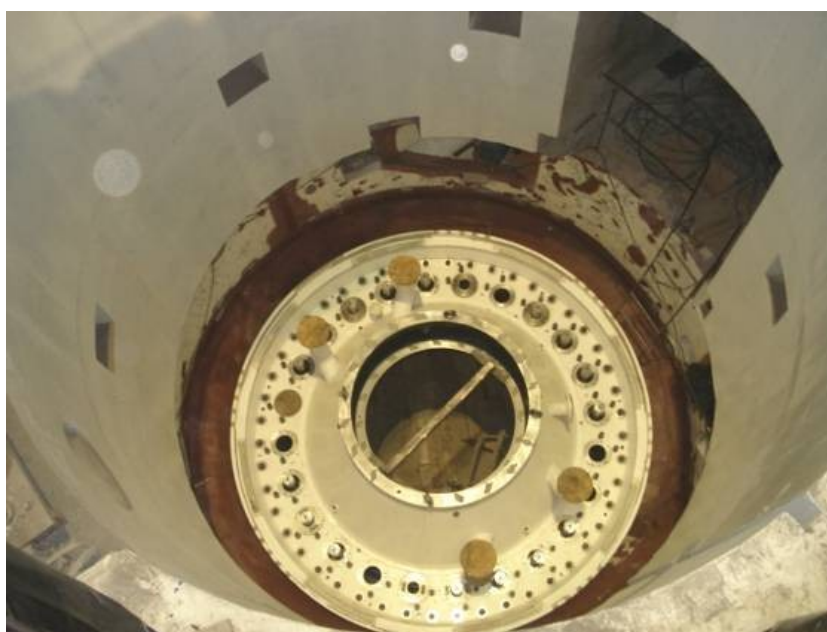
Figure 4.1 – Power House – Generation Unity 01 – Source: CERAN
