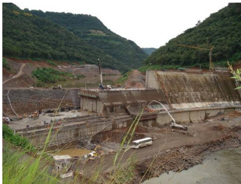
Figure 4.4 – Dam – Downstream General View – Source: CERAN
