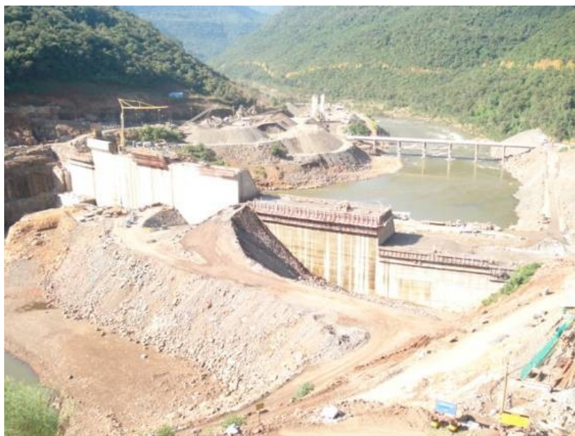
Figure 4.3 – Dam – Upstream General View – Source: CERAN
